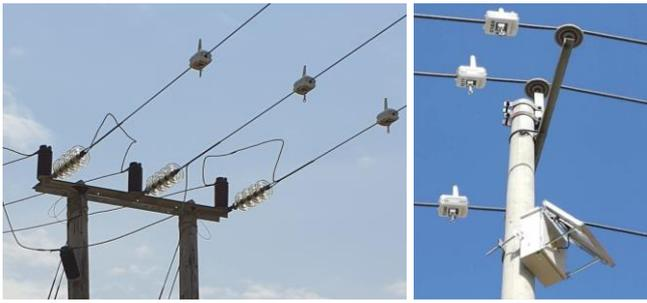
Fig. 1 (a) MetrySense 5000 sensors on an OHL (left) (b) Gateway unit installed on OHL pole (right)
