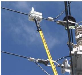
Fig. 6 Sensor installed using Grip-All hot stick
