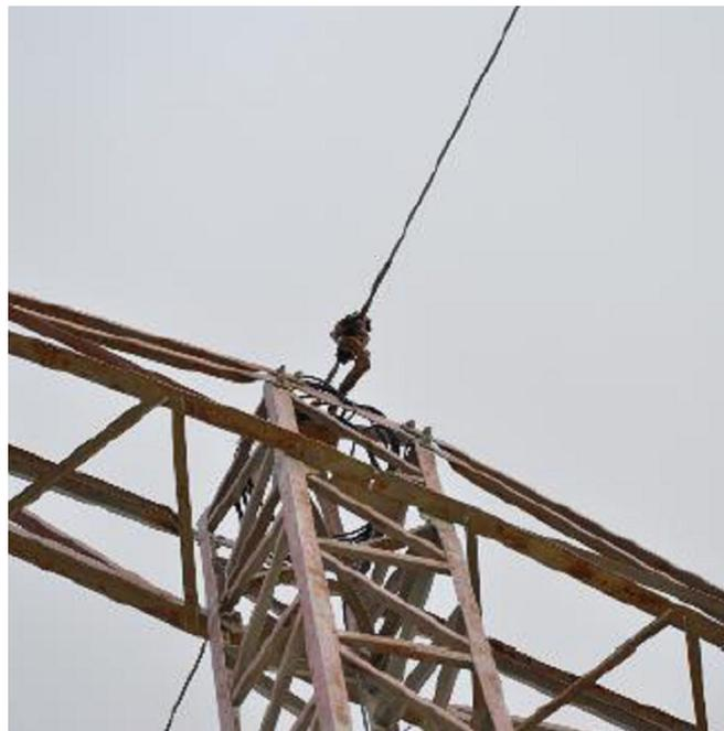
Fig. 8. Installation of the Sensor on the Shield wire
