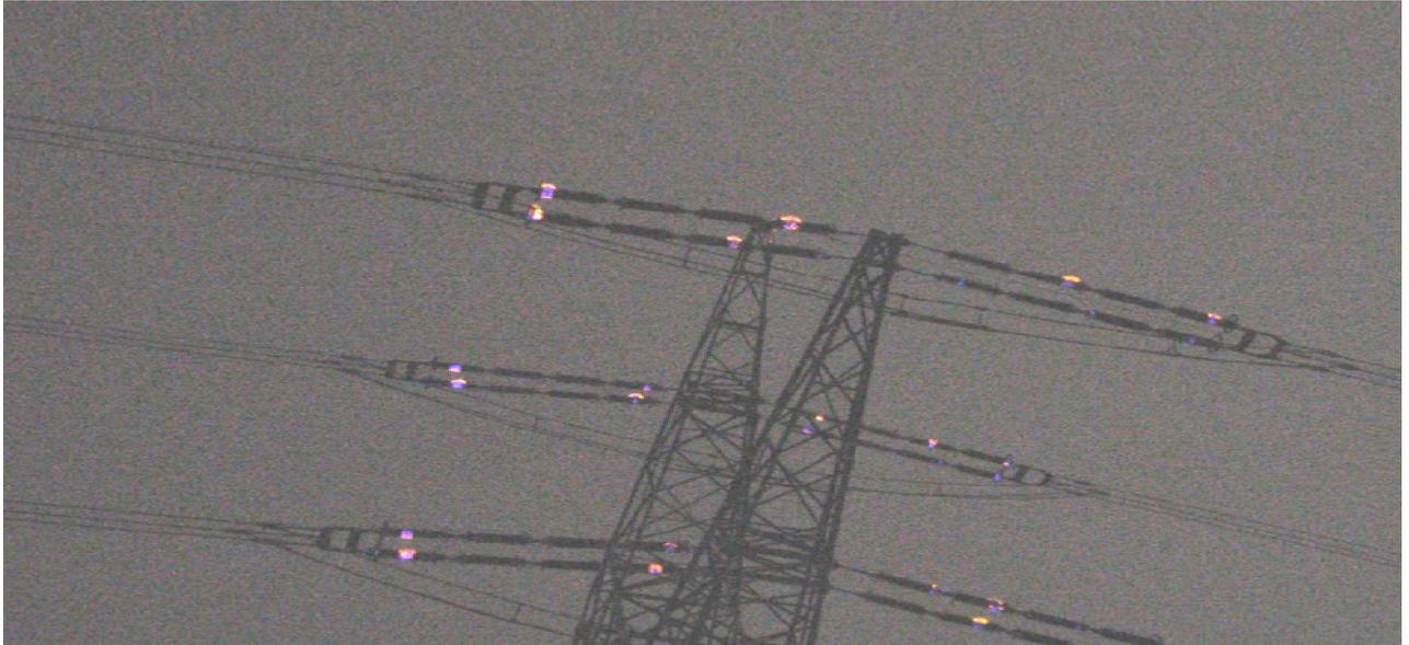
Fig. 1. Discharge on polluted insulators of a 400 kV line.
